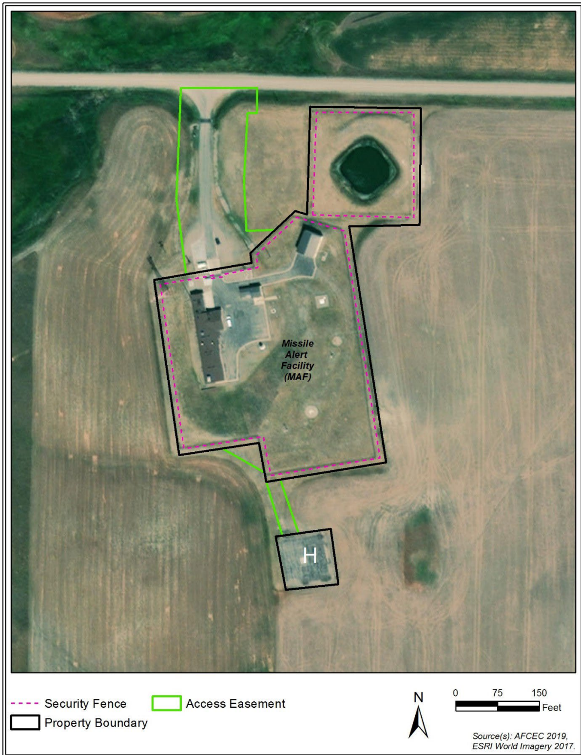
Figure 3. Aerial View of a Typical MMIII Missile Alert Facility
