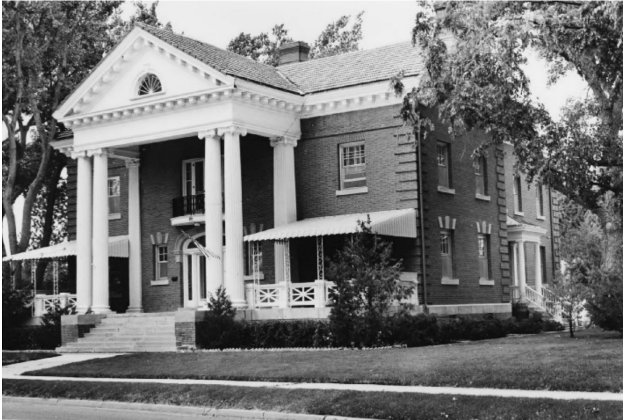
Figure 3.4-1. Commanding Officer’s Quarters, a component of the Fort D.A. Russell National Historic Landmark District on F.E. Warren AFB
