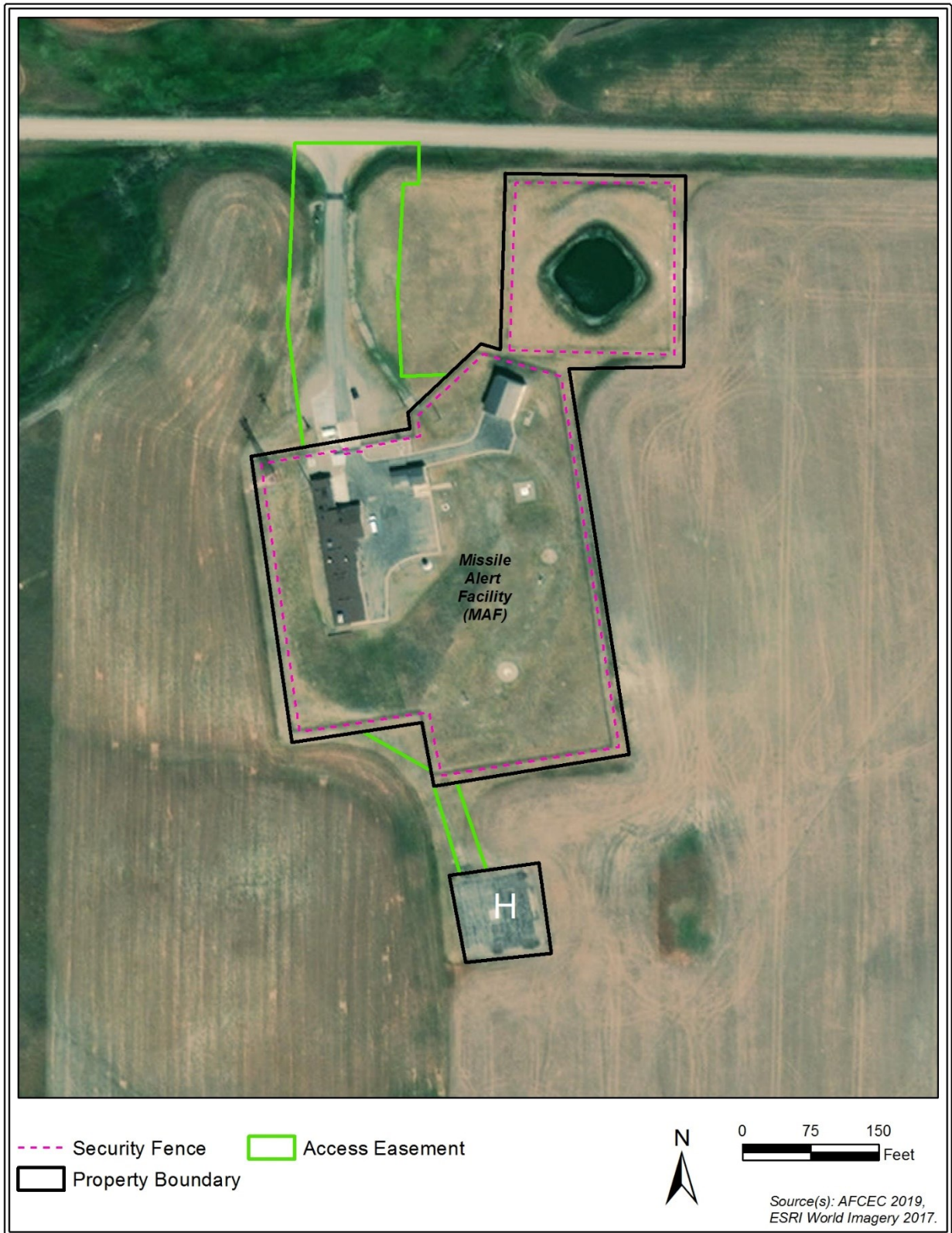
Figure 2.1-2. Aerial View of a Typical MMIII Missile Alert Facility
