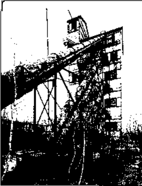
Building 561, Cannon Powder Blender, Picatinny Arsenal. Note the escape chutes to allow the workers to escape the building quickly. Source: HAER No. NJ-36C-83 , Picatinny Arsenal, Prints and Photographs Division, Library of Congress.
