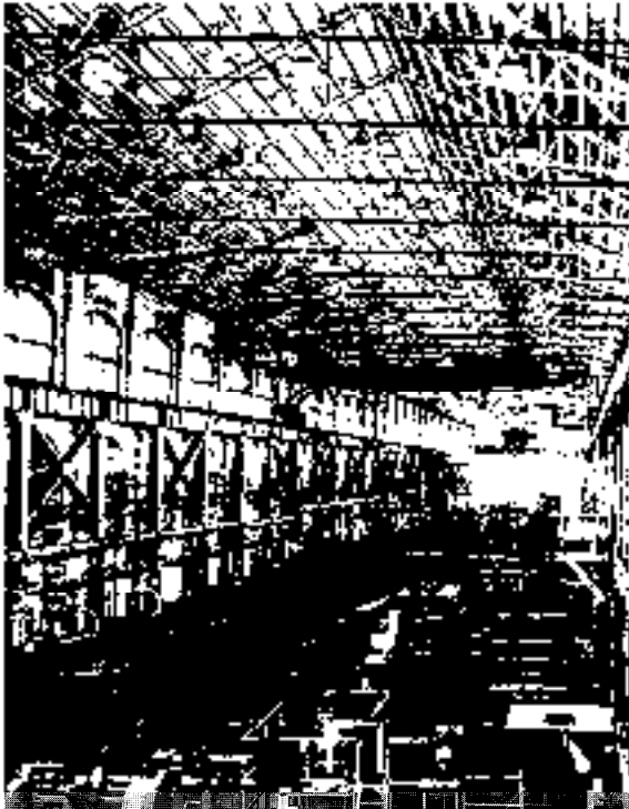
Interior view of the Big Gun Shop (Building 110), Seacoast Gun Shop, Watervliet Arsenal, 1985. Shown is the main bay with overhead cranes used for maneuvering the heavy gun tubes. Source: HAER NY-1 B-50, Watervliet Arsenal, NY, Prints and Photographs Division, Library of Congress.
