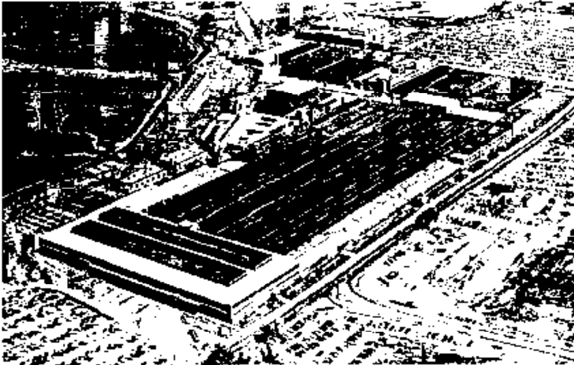
Air Force Plant 43 at Stratford, CT, ca. 1960. Compare this photograph to that of 1943 (first figure). Note the extensive additions, especially to the main assembly buildings at center. Also note the jet engine test cells at left center (at the base of the causeway). Source: HAER No. CT-14, Stratford Army Engine Plant, p 45, Prints and Photographs Division, Library of Congress.
