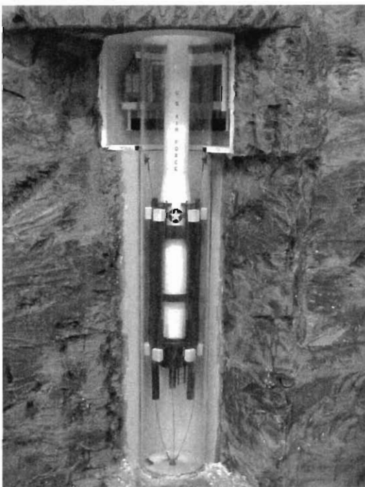
Cutaway of Launch Facility missile silo showing Minuteman II missile.
