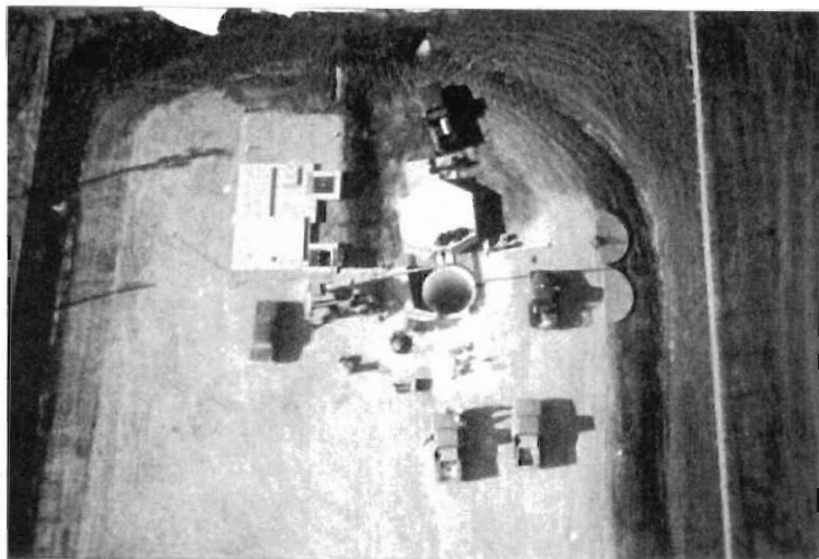
Launch Facility at Grand Forks, under construction.
