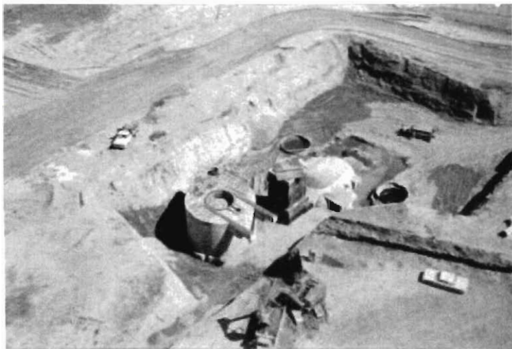
Launch Facility under construction in the mid-1960s.
